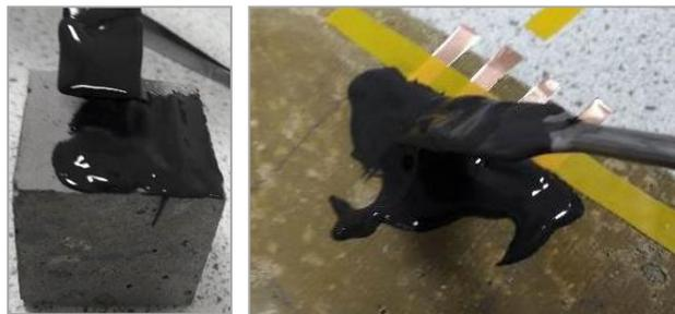
**Figure 10** – Procedure of putting geopolymer layers on concrete surface.
