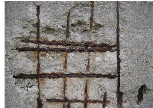
Figure 2 – Consequences of rebar corrosion.
