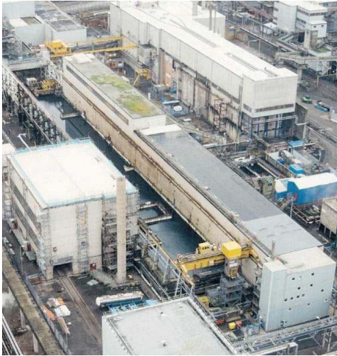
First Generation Magnox Storage Pond - Sellafield
