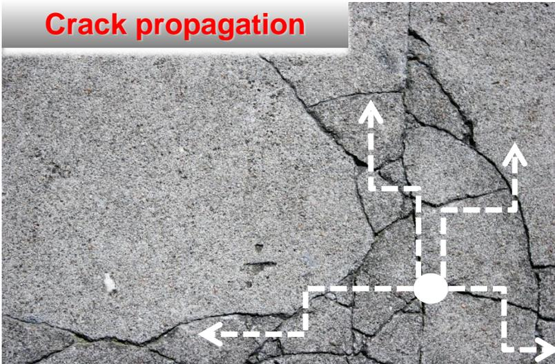
The main effect is the formation of **nano-micro-macro-dangerous** cracks. Those can in turn involve several reactions, increasing the moisture content, air entrainment, contamination flux and compromise the safety, standard conformity and workability of the concrete structures.
