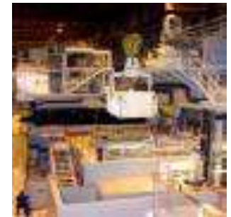
1 st Generation Magnox Fuel Pond
